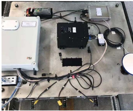
(b) 支持平台实物图 (b) Support platform of railway track vehicle
